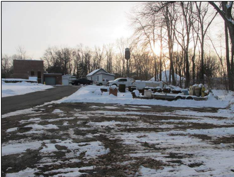
Photo 4: Looking south towards the headworks building. Proposed project site to the right.
