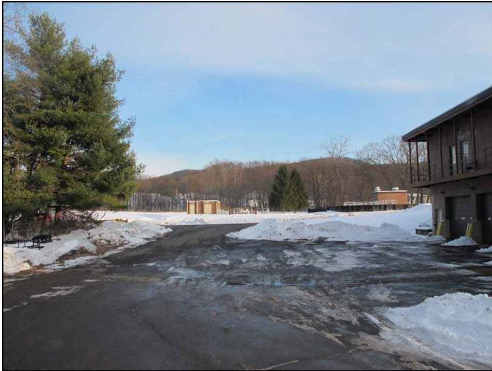
Photo 1: Behind the operations building looking east towards the sludge landfill and chlorination tanks.
