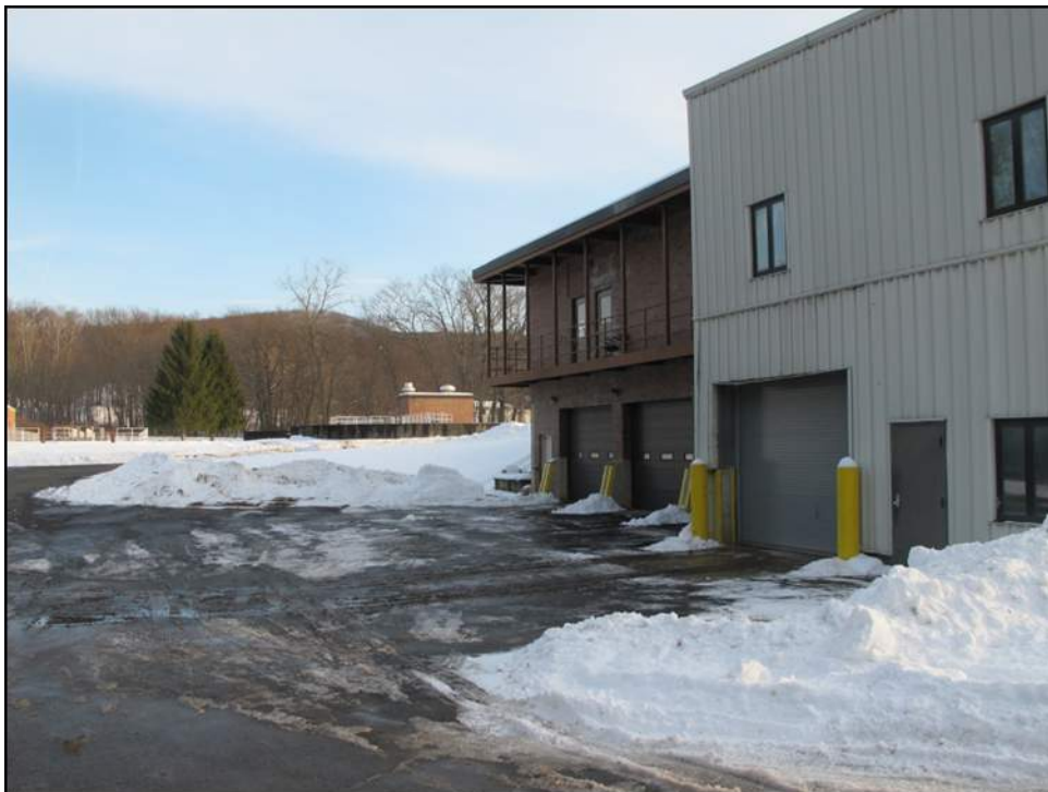
Photo 2: Rear of the main operations building.
