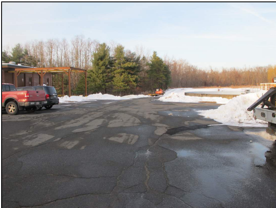
Photo 14: Looking north towards the existing sludge landfill.
