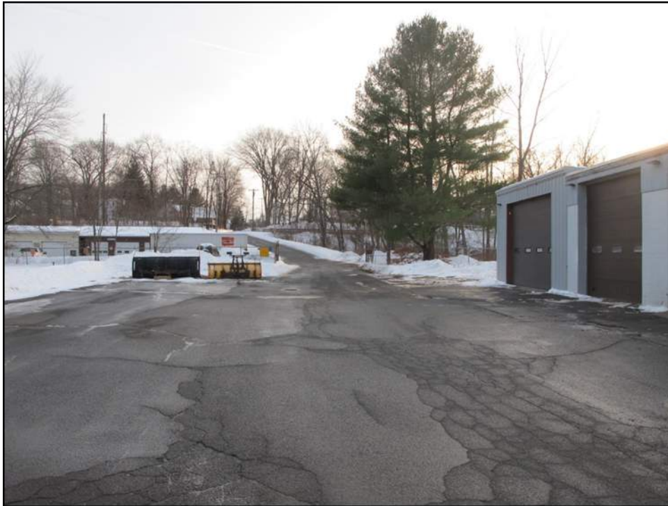
Photo 5: Looking south towards the main entrance of the WWTF.
