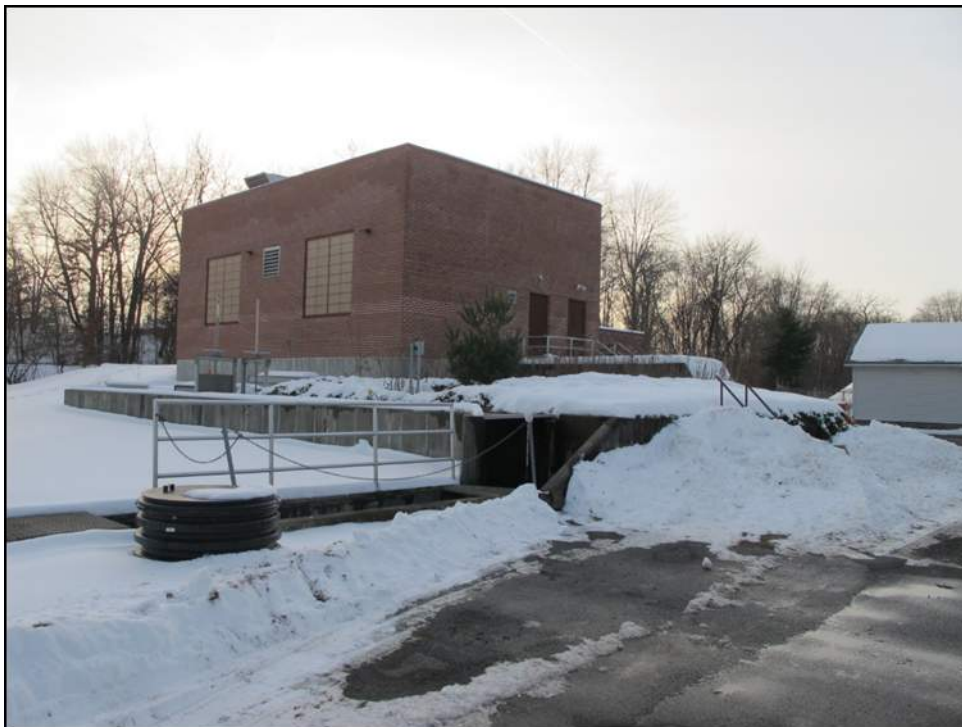
Photo 10: Headworks building at WWTF.
